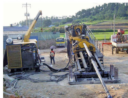
500 meters natural gas pipeline project in Weiyang Xi'an
