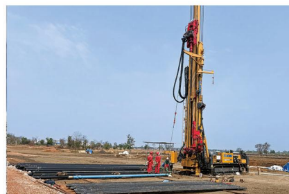
2000m water well drilling by Laos SINO-AGRI INTERNATIONAL
