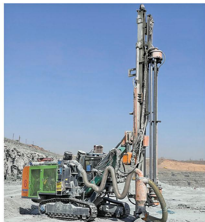
Blasting drilling in Ordos Coal Mine, Inner Mongolia
