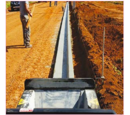
Automatic walking sensor, can correct direction, error within 1mm.
