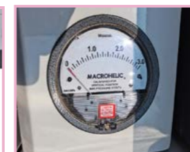
Pressure sensor controls filter element automatic cleaning
