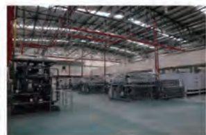
制粉车间 Powder Process Workshop
