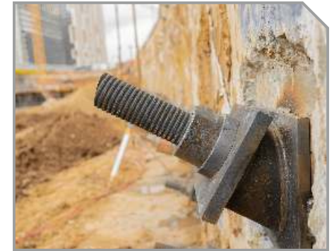
Installed ground anchor Atlant, residential complex «Sobytie», Moscow
