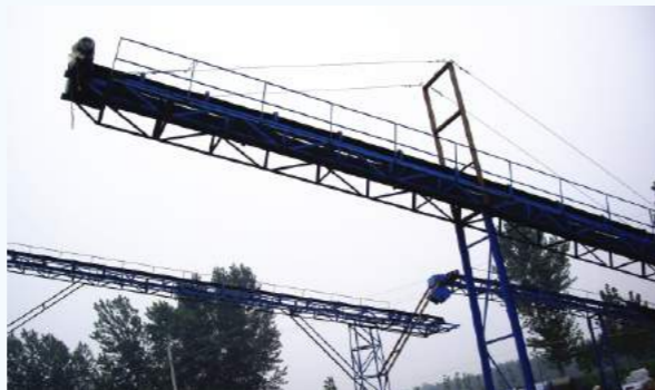
山东客户现场图 Customer Scene in Shandong
