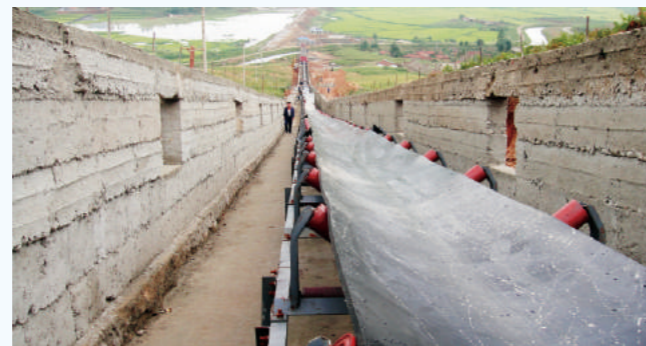
长距离输送机 Long-distance belt conveyor
