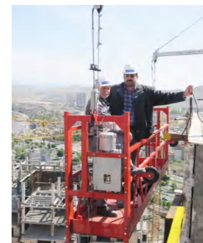
Curtain wall maintenance
