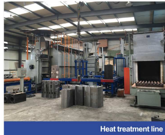
Heat treatment line
