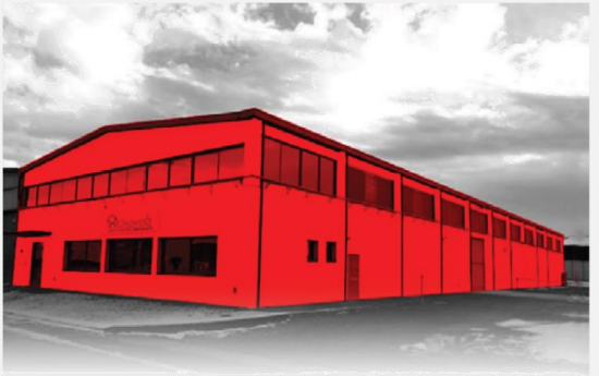
03 - Assembly & Testing plant ( 2.000 m 2 )
