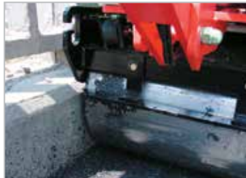
Low-Overhang for Compaction Right Up to the Edge of Curbside
