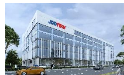
未来华东工厂在建 Future East China plant under construction
