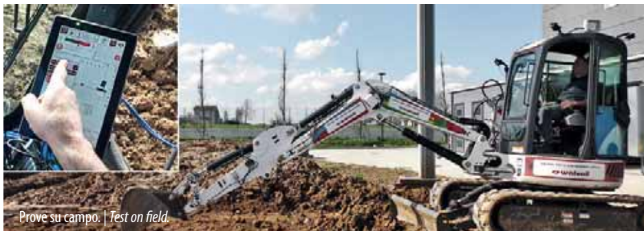
Nuovo Innovation Center Walvoil. | New Walvoil Innovation Center.
