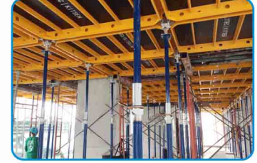
5 悬臂挂模 Climbing Formwork
