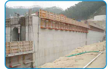
6 液压爬升模板 Self-Climbing Formwork
