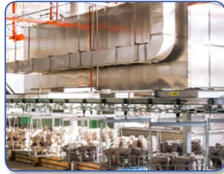
Automatic Shelling Pipeline
