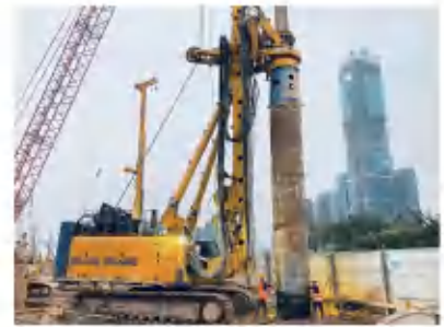
滨海大道(总部基地段)交通综合改造工程 Binhai Avenue (Headquarters Base Section) Traffic Comprehensive Transformation Project
