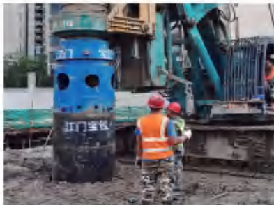
珠海斗门招商依云华府房建桩项目 Zhuhai Doumen Merchant Evian Huafu House Building Pile Project
