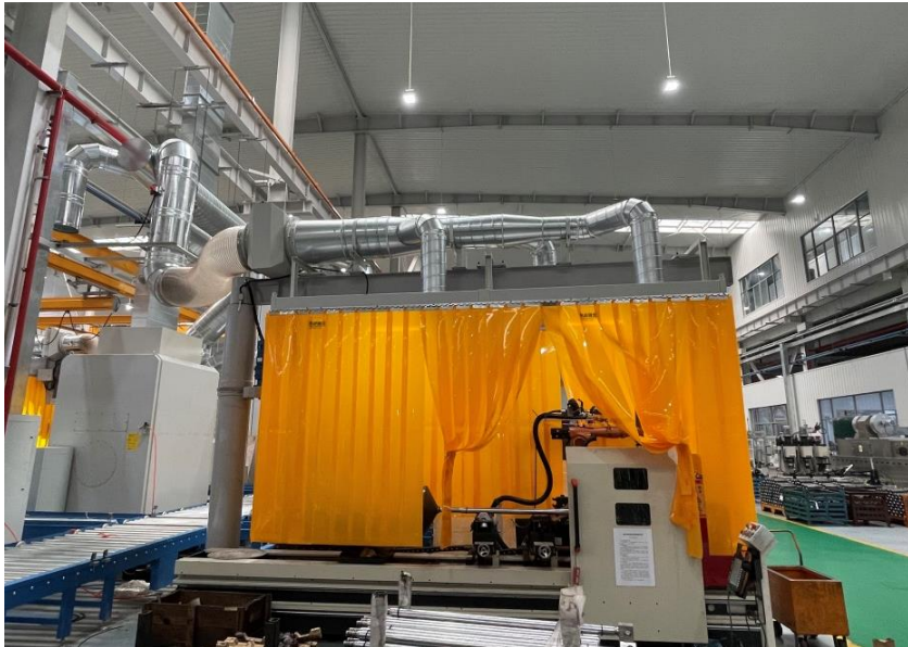
Welding robot for oil port
